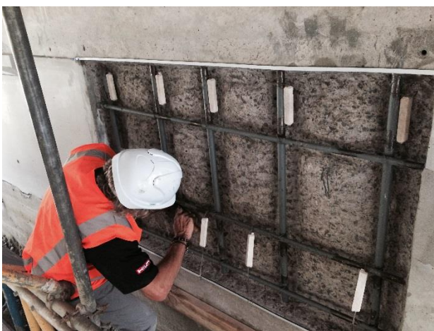
Cathodic protection to bridge piers affected by cracks, corrosion and spalled concrete, using embedded galvanic anode units 'Galvashield XPT' (left) and distributed galvanic anode system 'Galvanode DAS' (right)
