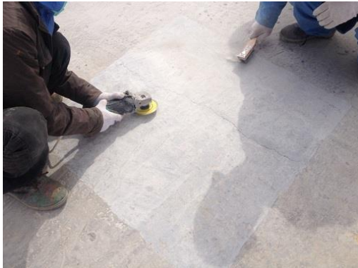
Linear Transverse cracks on new bridge deck due to plastic shrinkage- Surface grinding to open the face of the crack and sealing with epoxy resin
