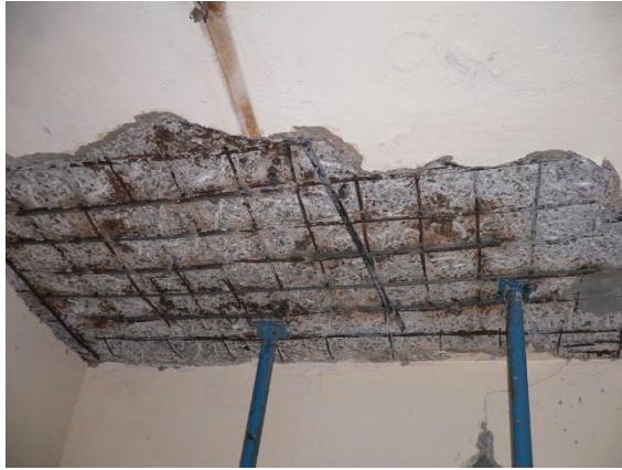
Soffits severely corroded due to roof leakages of a residential building
