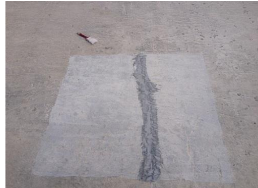
Linear Transverse cracks on new bridge deck due to plastic shrinkage- Surface grinding to open the face of the crack and sealing with epoxy resin
