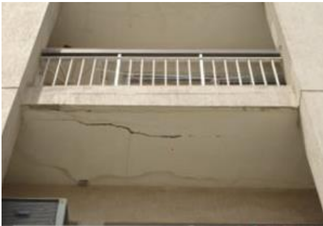
Balconies concrete corrosion and spalling due to multiple factors
