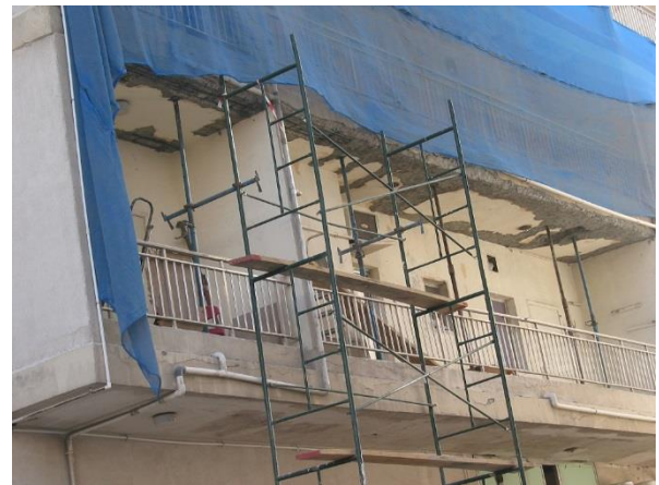
Balconies concrete corrosion and spalling due to multiple factors
