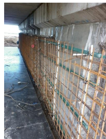
Cathodic protection to bridge piers affected by cracks, corrosion and spalled concrete, using embedded galvanic anode units 'Galvashield XPT' (left) and distributed galvanic anode system 'Galvanode DAS' (right)
