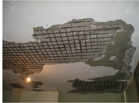
Soffits severely corroded due to roof leakages of a residential building
