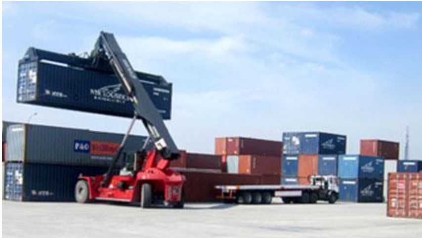
Container Yard: Capacity 400,000 TEUs per annum
