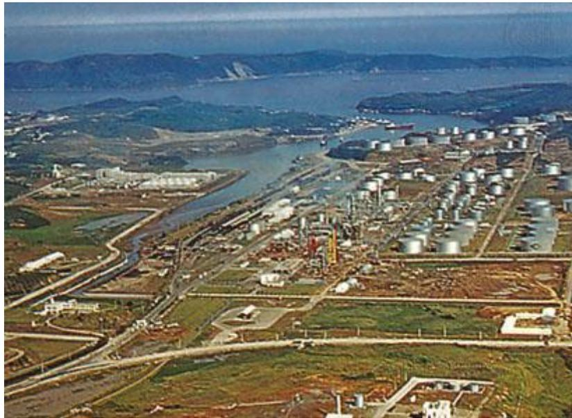
Opened in 1964, the Ulsan complex is the largest in South Korea and the second largest in Asia, housing 16 million barrels of oil in 34 large-scale crude oil storage tanks and producing LPG, Gasoline, Diesel, Jet Fuel and Asphalt for the foreign and domestic markets.
