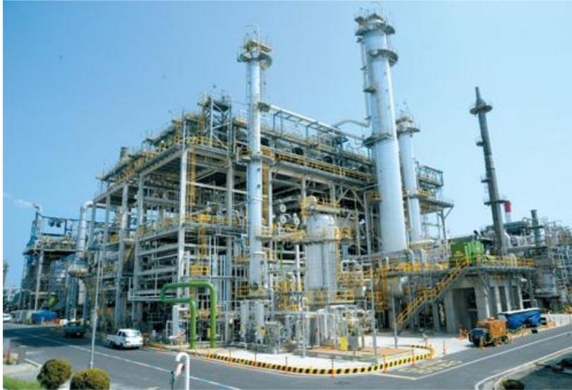
S Oil's Ulsan refinery complex is the South Korea's third largest refinery, and the second largest refining complex in Ulsan itself. The \$1.2 billion "Onsan Refinery Expansion Project" was completed in 2011, equipping the plant with an 89,000 bpd condensate splitter and petrochemical plants.
