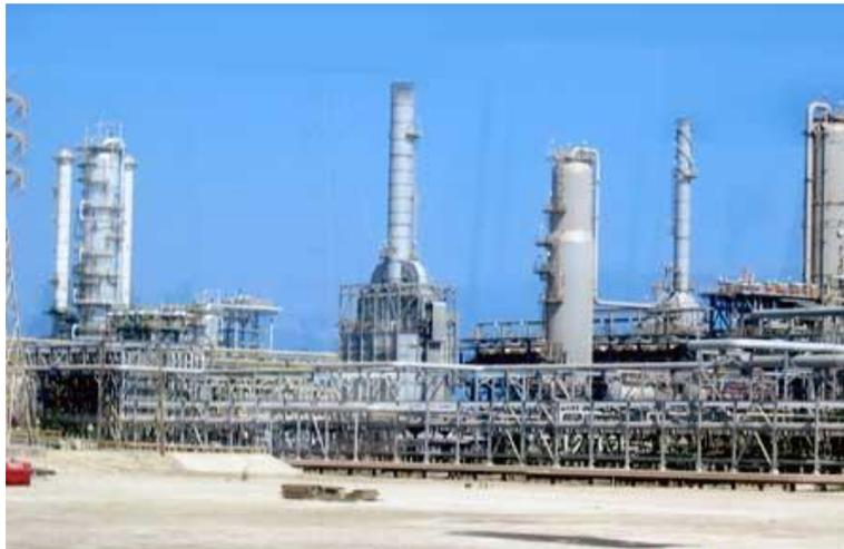
Ras Tanura is Saudi Aramco's largest refinery and the biggest in the Middle East. The complex processes both crude oil and gas condensates and has a natural gas liquids (NGL) processing facility and a crude stabilisation facility.
