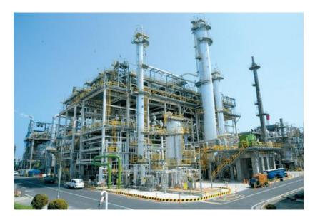
S Oil's Ulsan refinery complex is the South Korea's third largest refinery, and the second largest refining complex in Ulsan itself. The \$1.2 billion "Onsan Refinery Expansion Project" was completed in 2011, equipping the plant with an 89,000 bpd condensate splitter and petrochemical plants.
