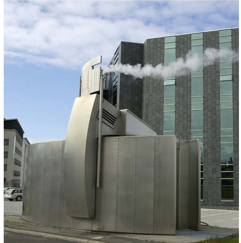
Completed wells ~ 5 * 5 m
