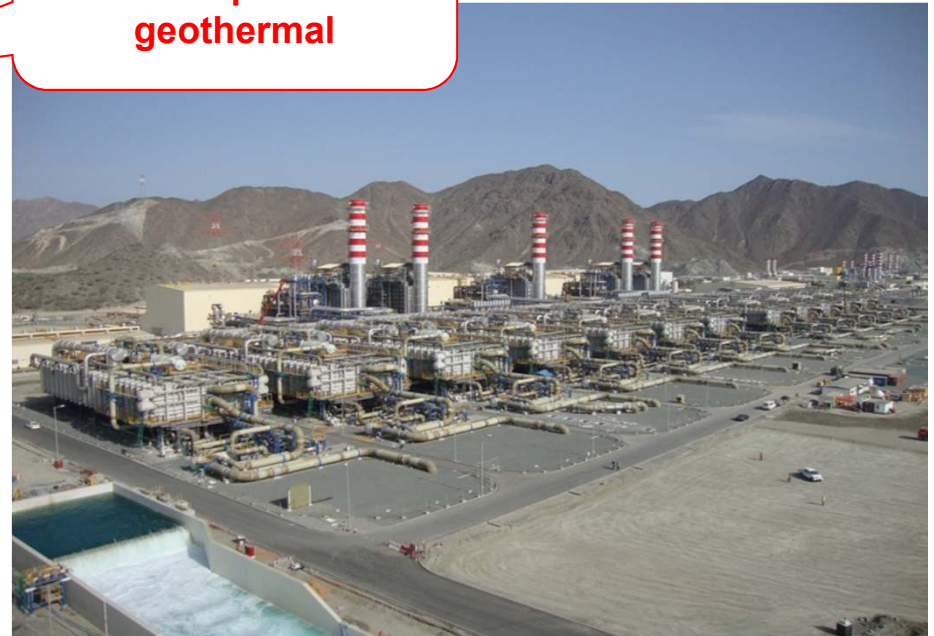
Fujairah II plant, UAE
