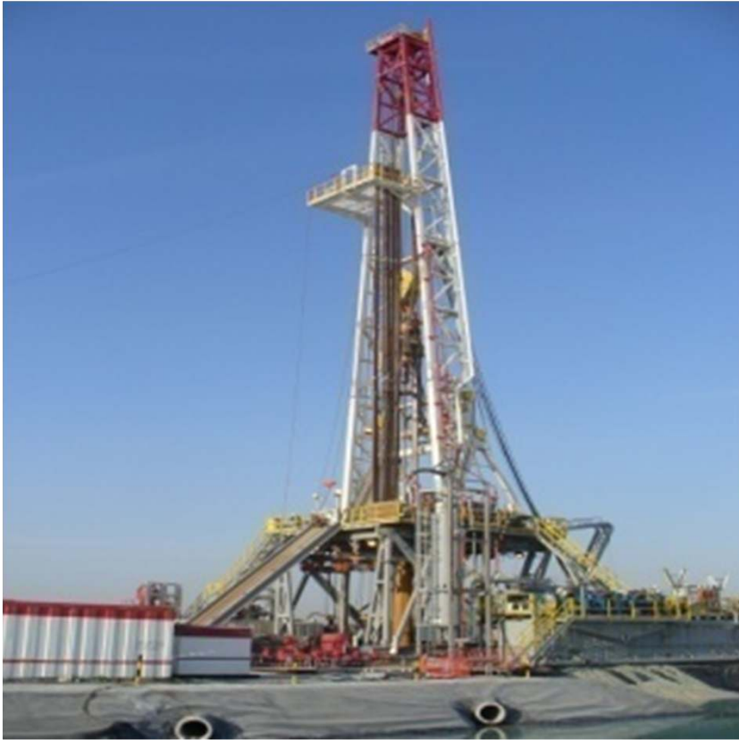
Well Drilling ~100 * 150 m
