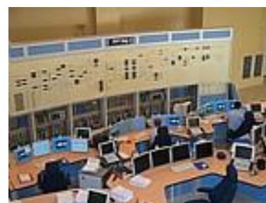
Computerised signal box
